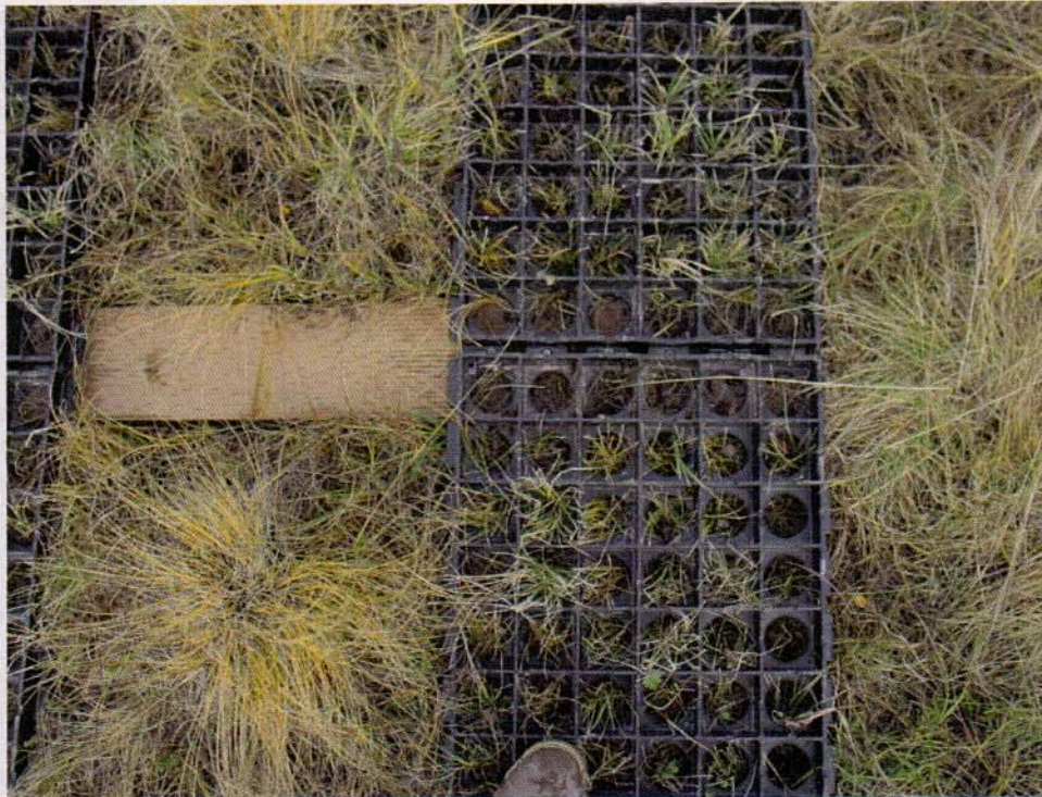
Photo 4. Detail of the cross tie joint. Note 1 5/8" deck screws fastened through the tab edge joints into the underlying 2X6 cross tie.
