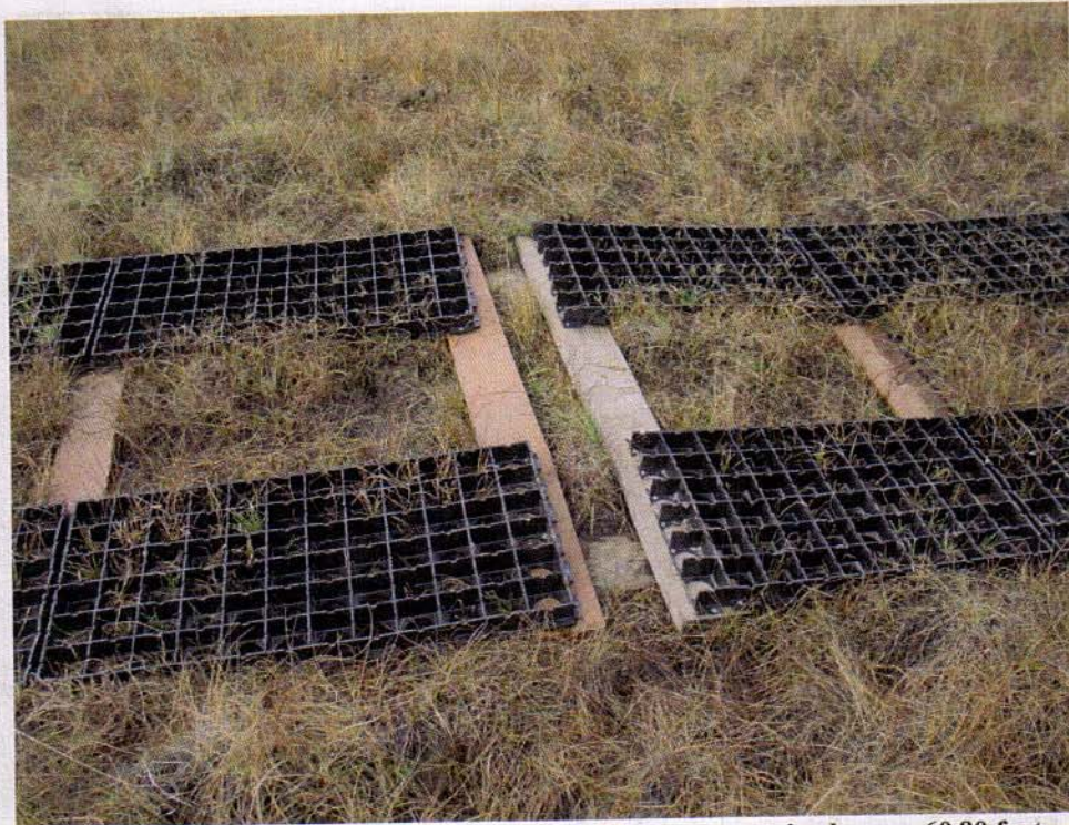
Photo 6. Detail of a thermal expansion joint. These are required every 60-80 feet along the installation to provide for panel shrinkage and swelling. Note use of 2X6 skid plate under panel-end cross ties. The gap (approximately 6 inches) between the panels is easily crossed by ATVs.
